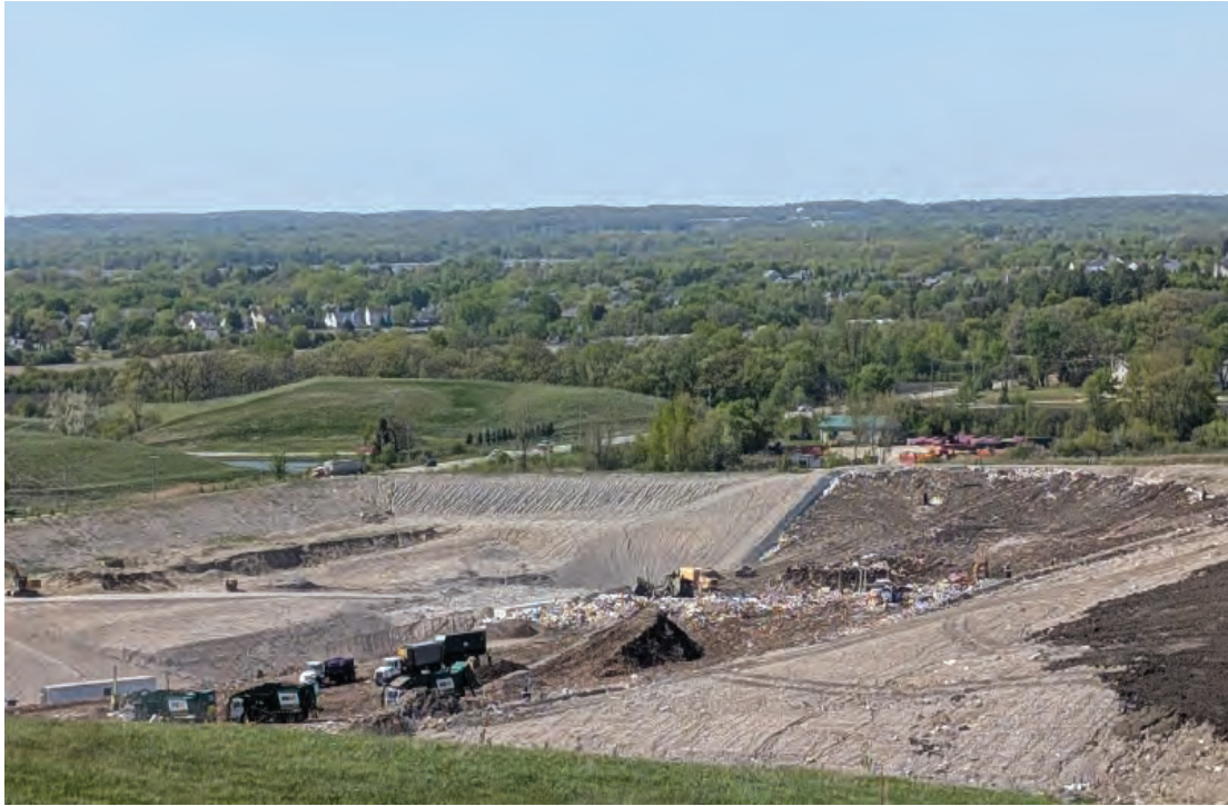
North end of Phase 4, needs covered
