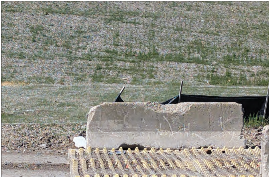
Rumblew mats for cleaning tires on site exit
